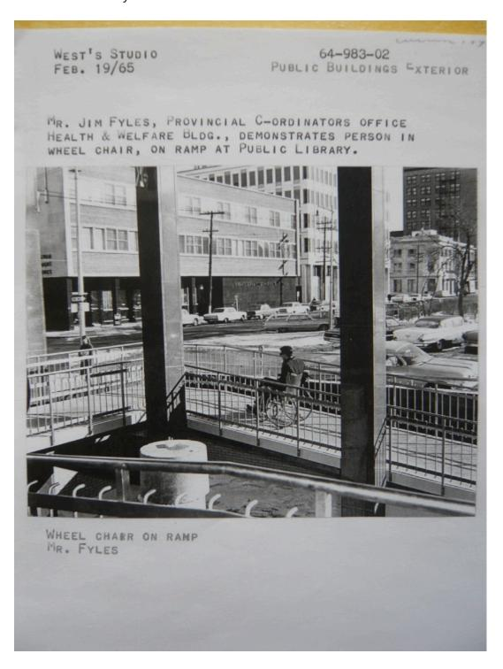
The guardrails, now 1.5 centimetres too low, they were to code in 1962, and they are elegant. Are the rails now too low because the concrete has been repaired? At one point, a lumpy asphalt coating was added, making it difficult for a wheel chair to even get onto the ramp. A 1.5 cm difference (2/3 inch) of beautiful aluminium hand rail should not give cause to tear down a building.
